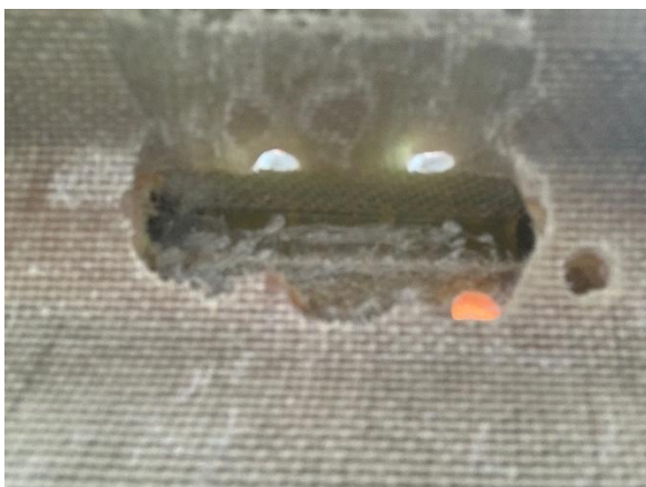
Showing the hole to allow access to the nuts & bolts
